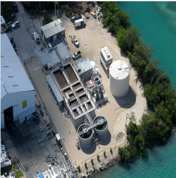
Duck Key Wastewater Treatment Plant Improvements
