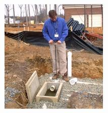
Fairfax, Virginia requires all new and repaired individual wastewater systems to install a flow diversion valve, like this one pictured, to allow the drainfield to dry out and avoid saturation problems.
